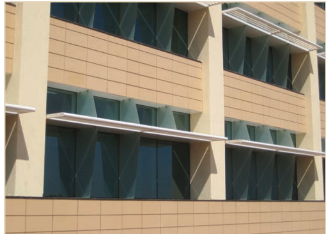
FIGURE 2: South façade sun shading and lightshelf detail, full daylight, no direct solar or glare.
