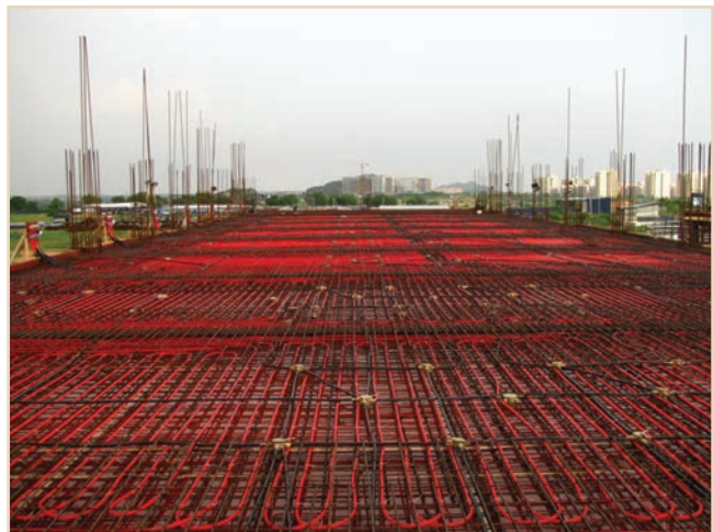
FIGURE 6: Radiant slab system before concrete pour.
