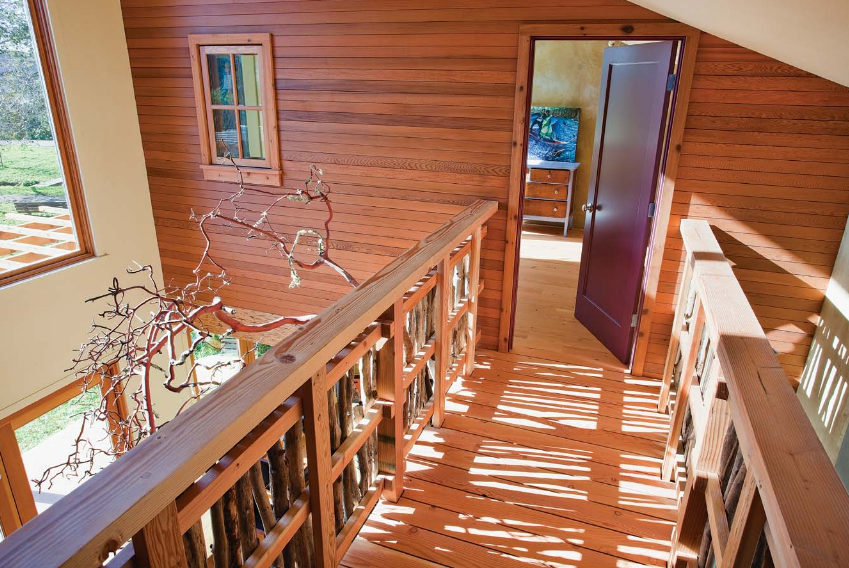
Bridge to bedtime. The bridge offers a bit of privacy by separating the master bedroom from the kids' rooms, and the open two-story space and interior windows in all the bedrooms allow sunlight to flow freely through the second floor to spaces below. Photo taken at G on floor plan.
