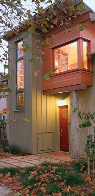
Material palette found. A driftwood column welcomes guests and supports the cedar-clad bump-out above. Straw-bale walls are finished with lime plaster while board-and-batten fiber cement marks the stick-framed stairwell. The front door and interior windows are Craigslist finds. Photo taken at C on floor plan.
