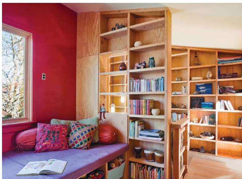
Double-duty framing. In the stairwell, the interior walls are used for bookcases. A bump-out built-in turns the hallway into a play area. Photo taken at H on floor plan.
