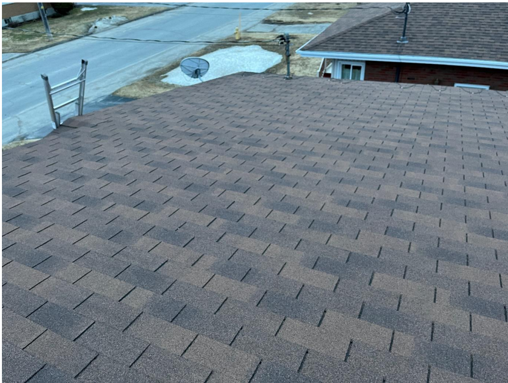
Left side of roof looking from roof peek.
