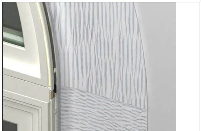
Figure 10: Use flexible flashing for radius head jambs
