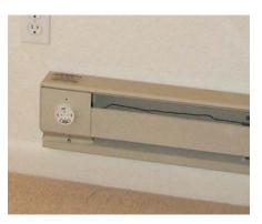
The heating element in an electric baseboard unit works just like the element in a toaster. Any electrician can install these units fairly quickly. The main drawback to this solution is that in most areas of the country, electric-resistance heat is expensive to operate. Still, electricity costs vary widely in the United States, from a low of about 6¢ per kwh to as much as 20¢ per kwh. The lower your electricity cost, the more attractive electric-resistance heating becomes.
